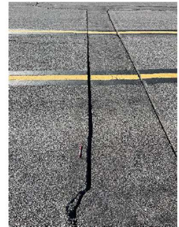
Patch failure on Runway 8-26
