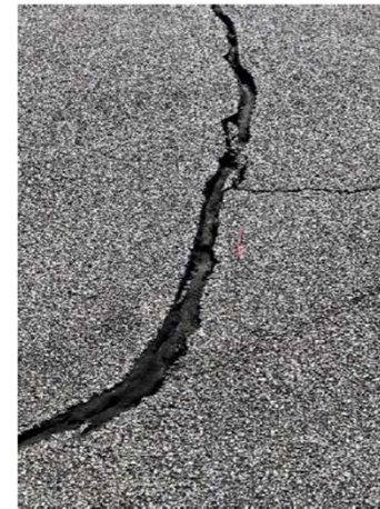
Transverse thermal cracking on Runway 8-26
