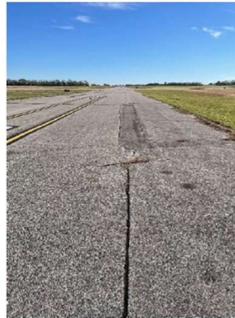
Longitudinal cracking on Runway 8-26
