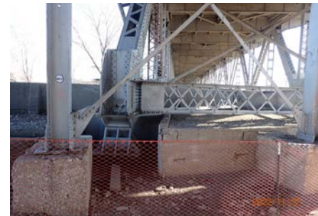
Image 5: Repairs underway on main river span truss bearing
